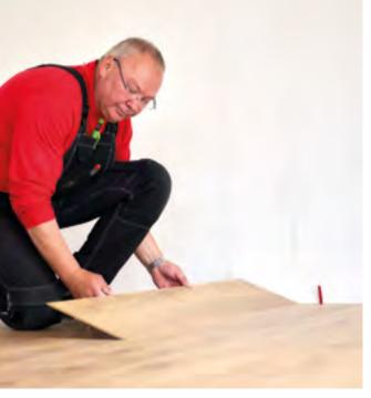
The click system makes KRONOTEX laminate easy to lay. Clothes pins help with the distance from the wall.
