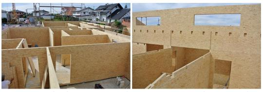
Rapid assembly of prefabricated elements (photograph: BALAZS Komforthaus GmbH)
